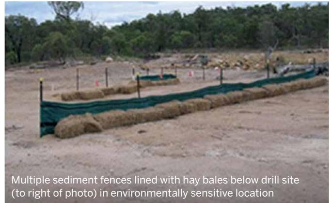
Multiple sediment fences lined with hay bales below drill site (to right of photo) in environmentally sensitive location
