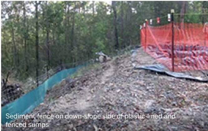
Sediment fence on down-slope side of plastic-lined and fenced sumps
